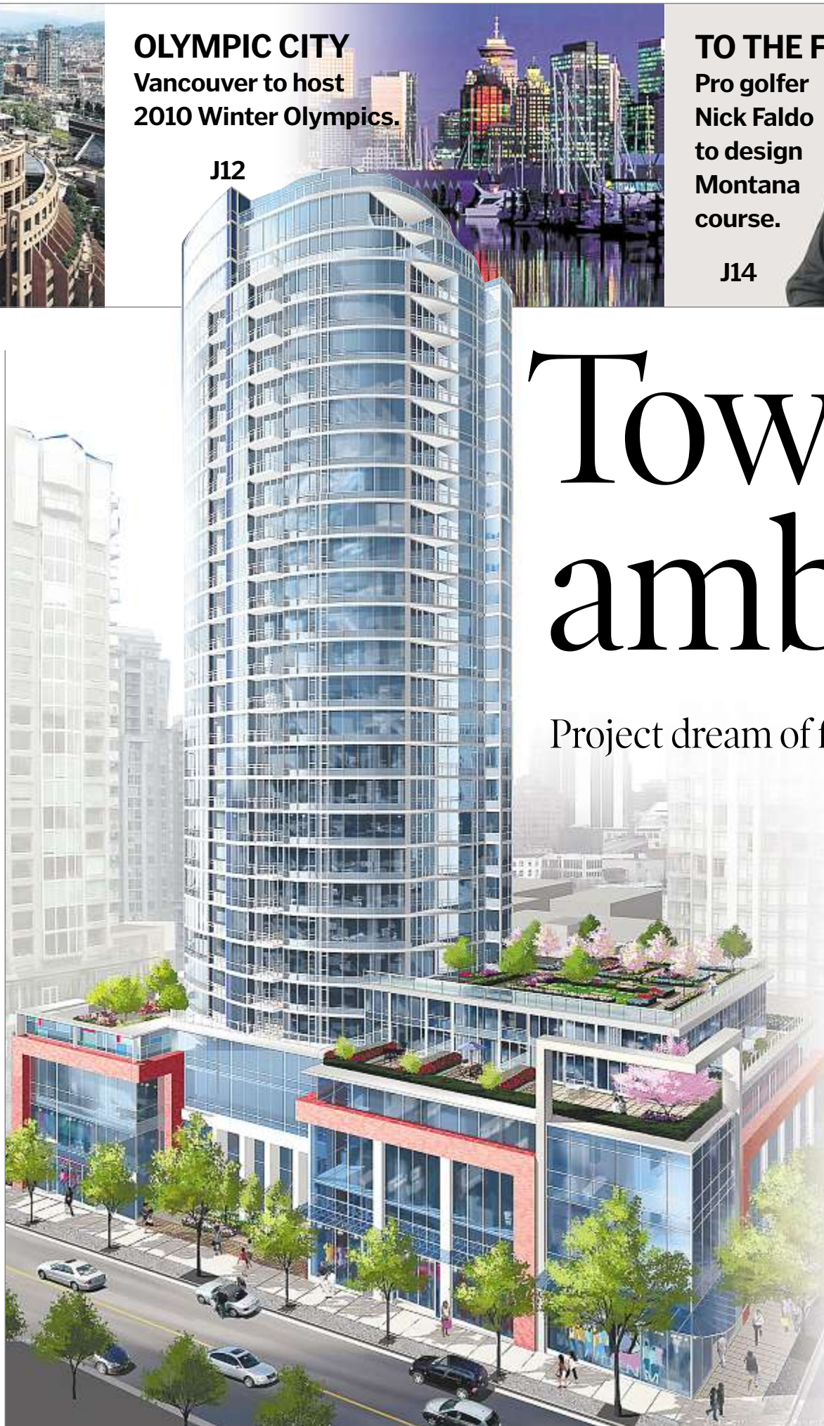
The Atelier is a sleek, modern highrise condo tower slated for Robson Street in Vancouver.
